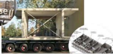
Figure 36 - Examples of harvested materials from the 10-story housing block (on building, product and material level) to be used in new construction (Düsseldorf 2019).
