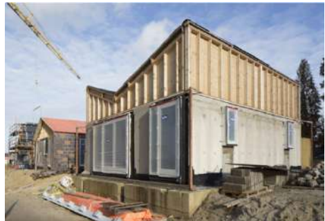
Figure 36 - Examples of harvested materials from the 10-story housing block (on building, product and material level) to be used in new construction (Düsseldorf 2019).
