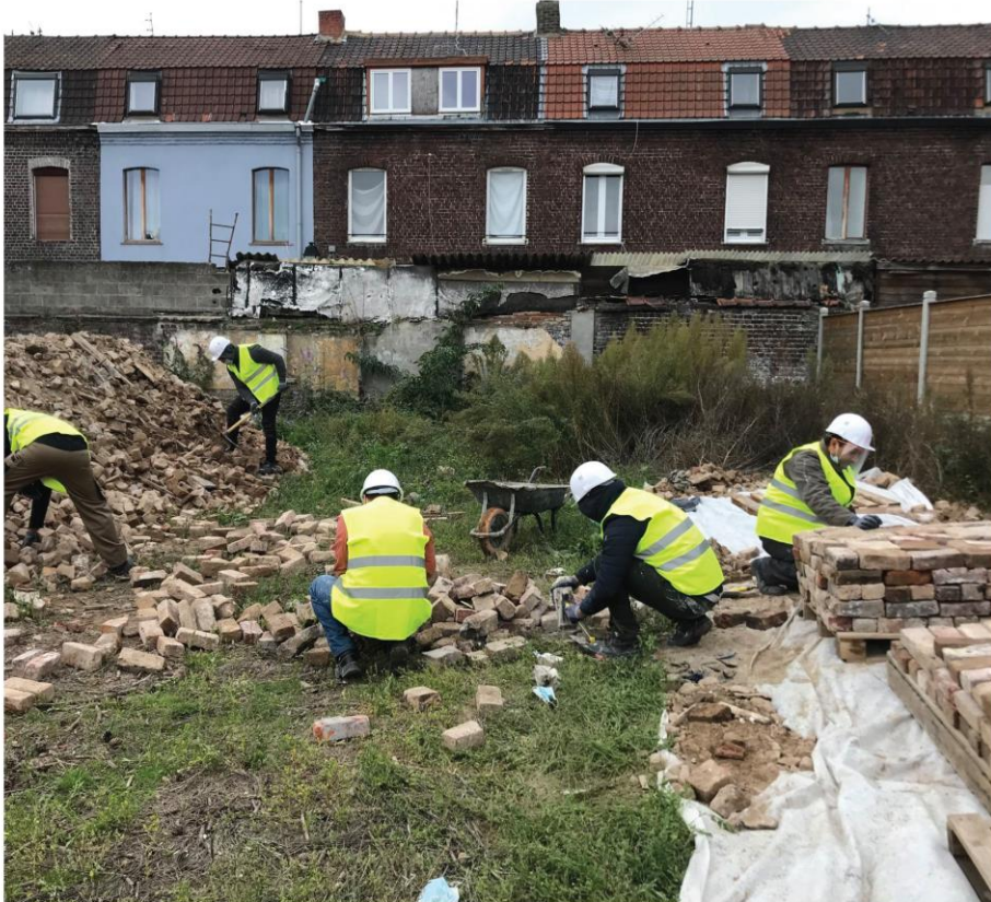
Recovering of bricks from a demolition work © La Fabrique des Quartiers
