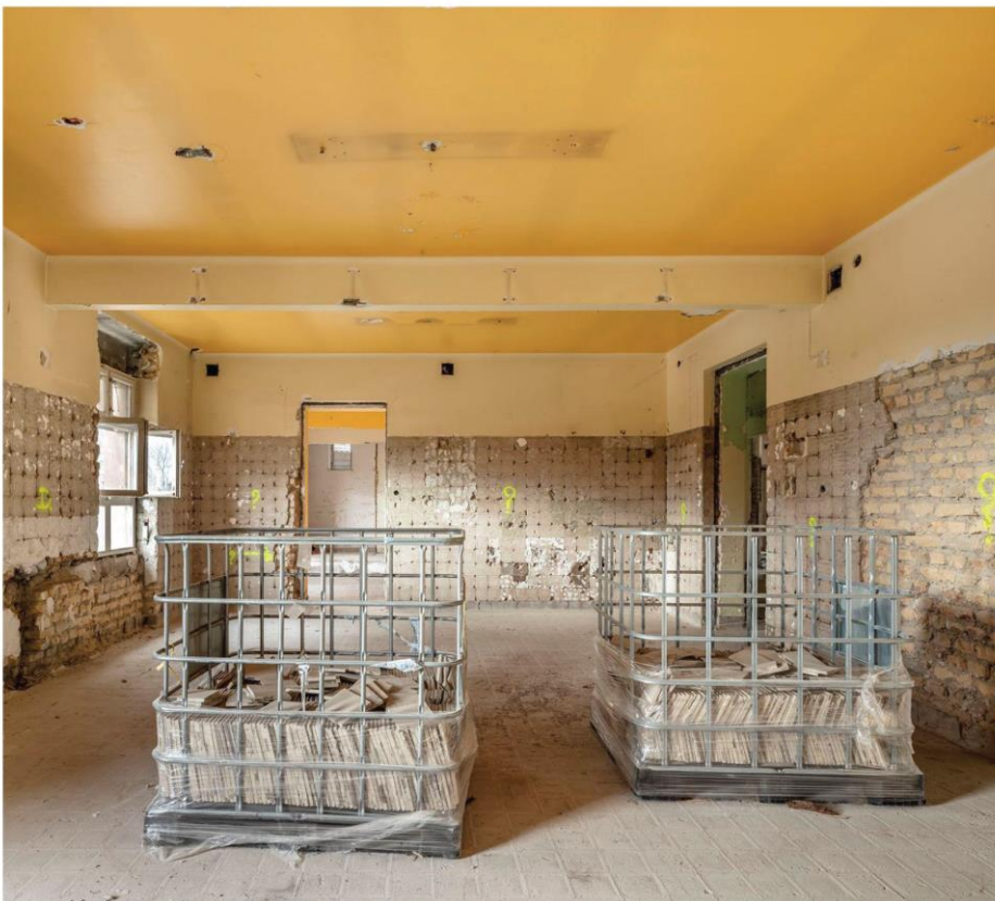
Dismantled tiles, packed for transport © Luc Boegly
